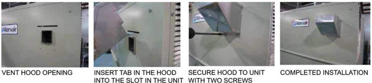
Figure 9. Vent Hood Installation
